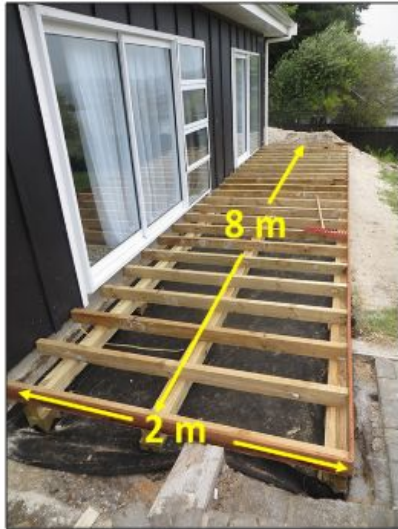
Deck measuring 8 metres \times 2 metres
